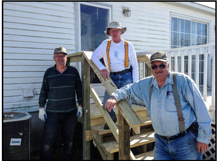
The work crew: Bob, Jim, Herb, Mike Quinn (not pictured).
