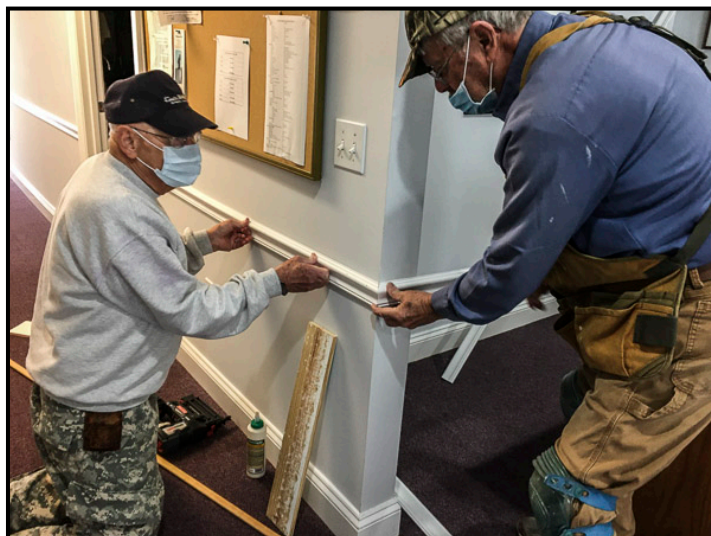
Installation of chair rail in Memorial Hall
