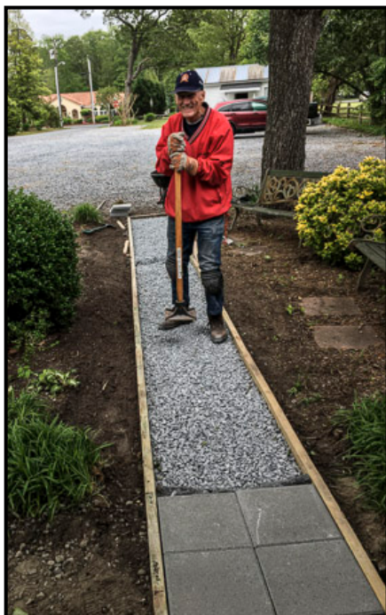
Sidewalk remodel continues.
